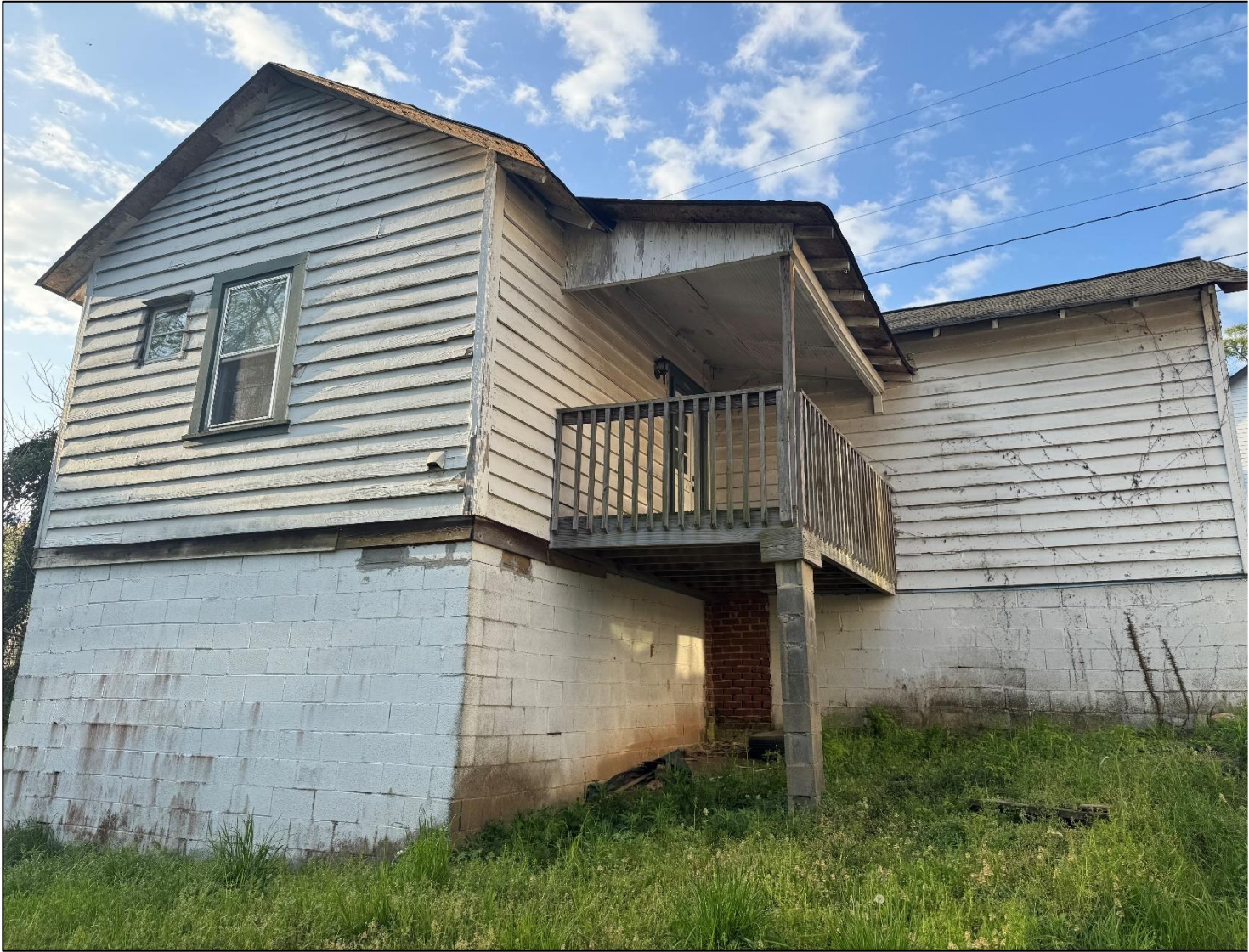
Figure 5. Existing rear façade at 55 Maple Street (photo from Staff)
