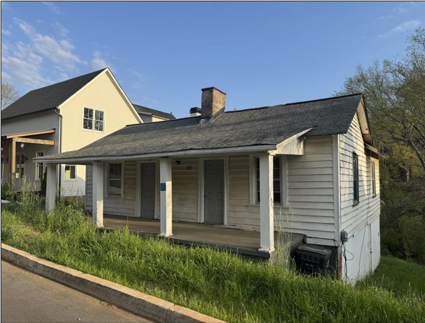
Figure 1. Existing front façade of 55 Maple Street (photo by Staff)
