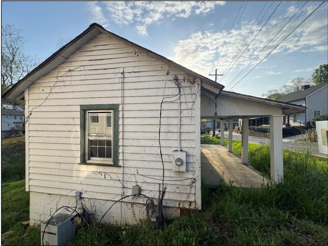
Figure 2. Existing left side façade of 55 Maple Street (photo by Staff)
