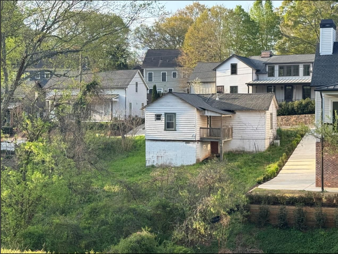
Figure 3. Existing rear facade at 55 Maple, as seen from Oxbo Road (photo from Staff)
