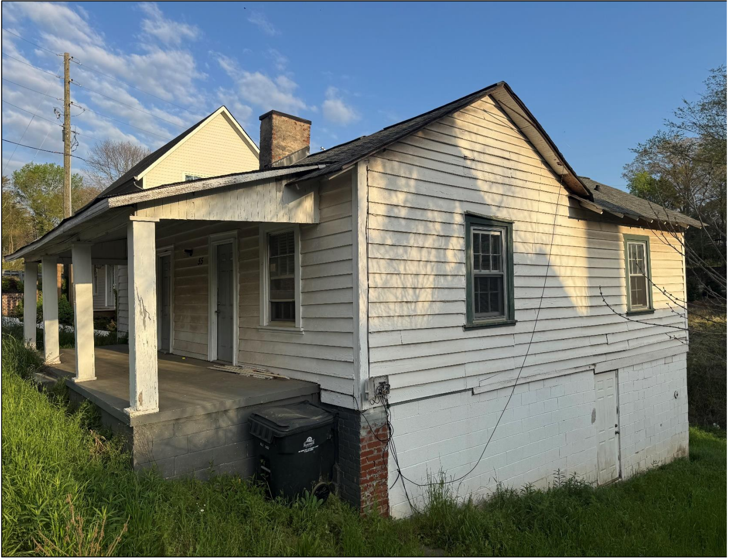
Figure 4. Existing right side façade at 55 Maple Street (photo from Staff)
