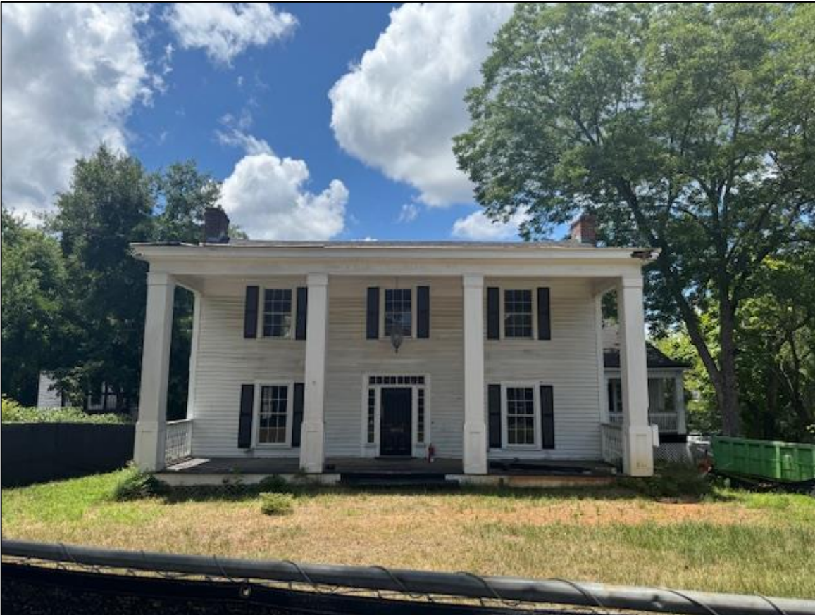
Figure 2. The existing front façade of Founder's Hall/1076 Canton Street (photo from Staff)
